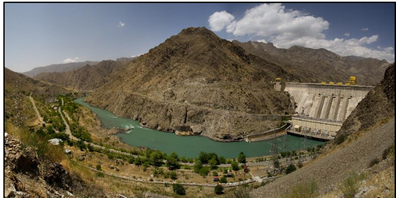
The Kurpsai Dam on the Naryn River in Kyrgyzstan (Source: Photo by Hy AlgeriaK; Wikipedia)
